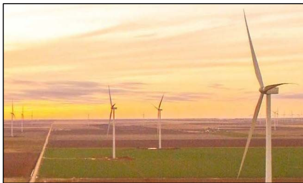
Fort Hood, Texas: 65 MW AC Hybrid Wind & Solar Projects; Expected to provide $100 million in cost avoidance over the term of the 30-year contract
